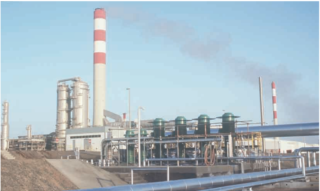
Rabigh Refinery. Courtesy of Saudi Aramco.
