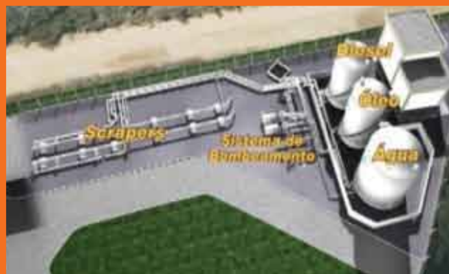
12" diameter - 2.4km in length with integral supply tanks, pumps, automation and state-of-the-art controls.
