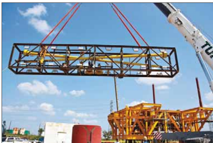
Hoisting the components of the subsea electrical pump.
