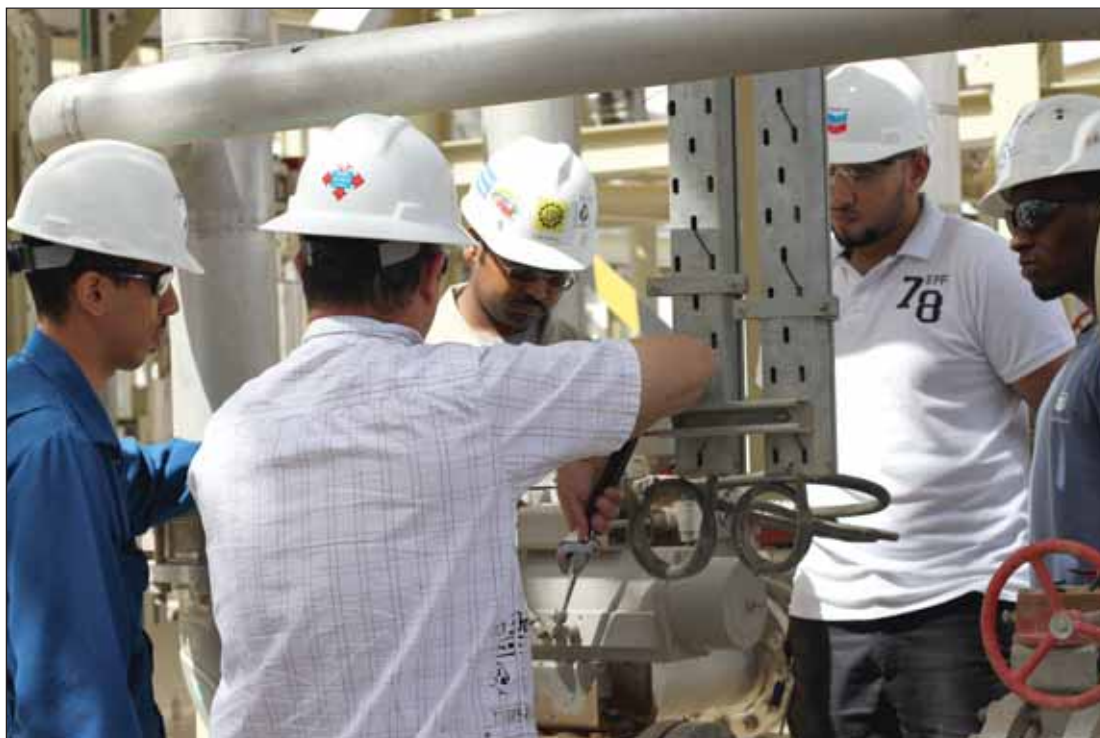
LSP autotechs and operators troubleshoot an electric control valve actuator for process water for the LSP water plant.
