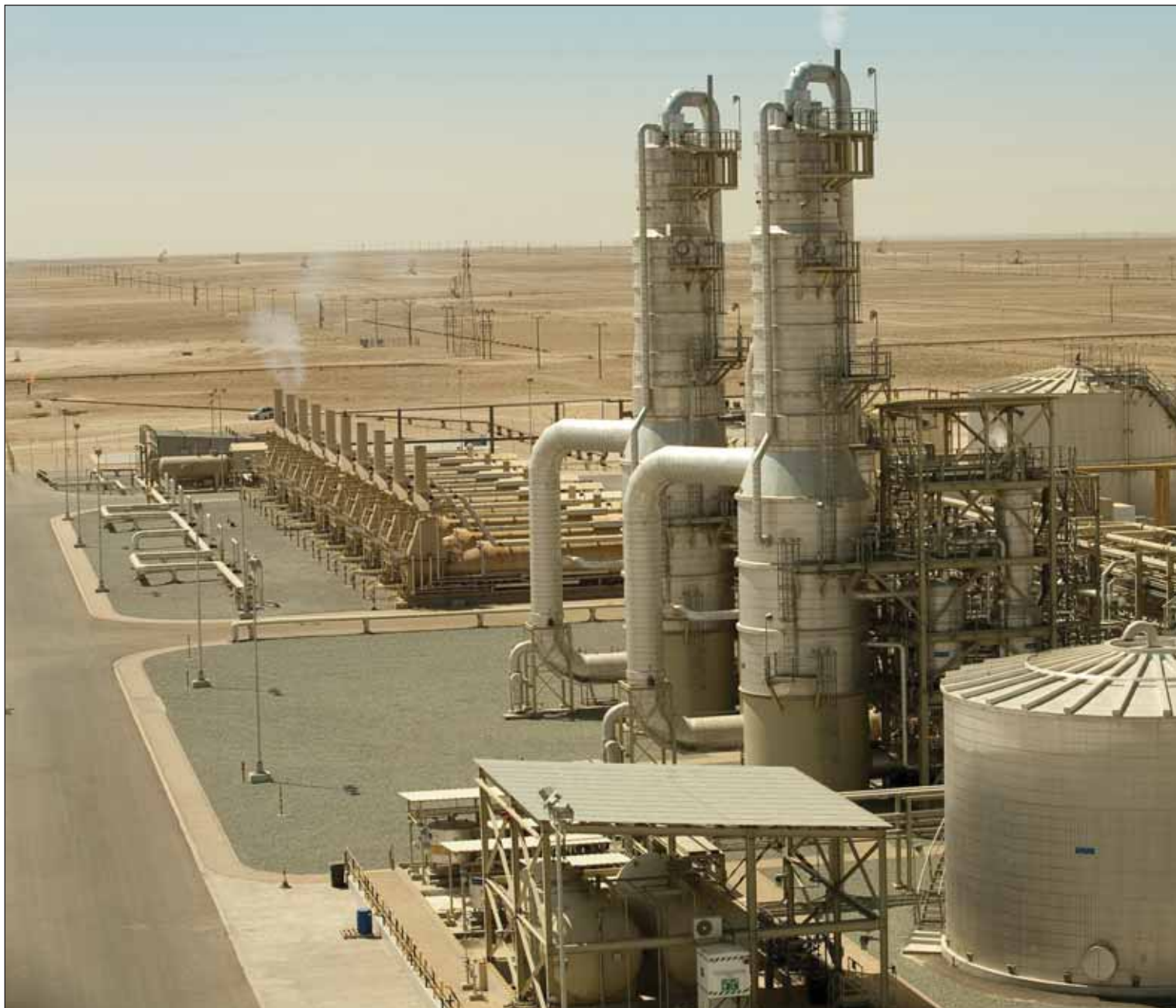
Produced water is cleaned to a high purity in the two evaporators of the water plant for the First Eocene Large Scale Pilot before being converted by its 10 steam generators into high purity steam for injection in the field's First Eocene reservoir.
