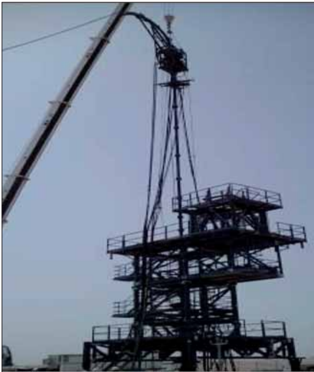
Fig. 8. CT tower rigup during deployment/reverse deployment.
