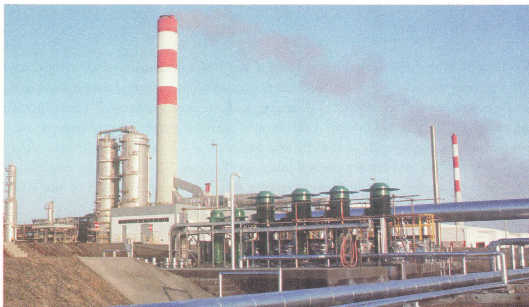
Figure 6 - Rabigh Refinery (Courtesy of Saudi Aramco)
